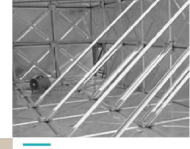
There are 4 different types of metal stays with two different classification, this is best described as tiers 1 to 4 and either triangular or horizontal - Tiers 1 and 2 are manufactured out of 70 x 70 x 6 angles with 8 mm base plates and tiers 3 to 4 are 60 x 60 x 6 with the same 8 mm base plate
